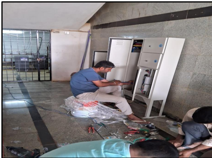
Fig:2 Connecting Solar Panel to Grid
